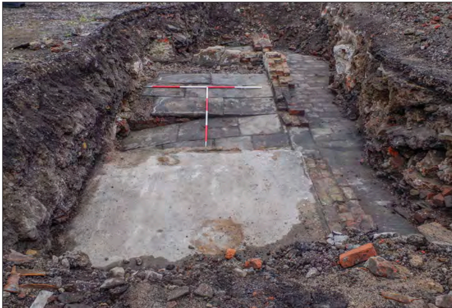
Plate 70: Overview of trench 11 slaughterhouses from west showing concrete floor repair 11017 (foreground), the fall of floor 11015 (under scales) and black ash mortar repair 11007 (right of scales)
